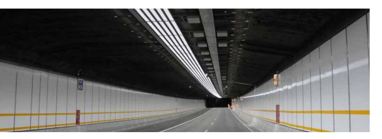
The superior colour rendering and higher perceived brightness makes it easier to distinguish objects and shapes. Drivers detect movement faster and from a greater distance with white light, giving them more time to react should the unexpected happen.
