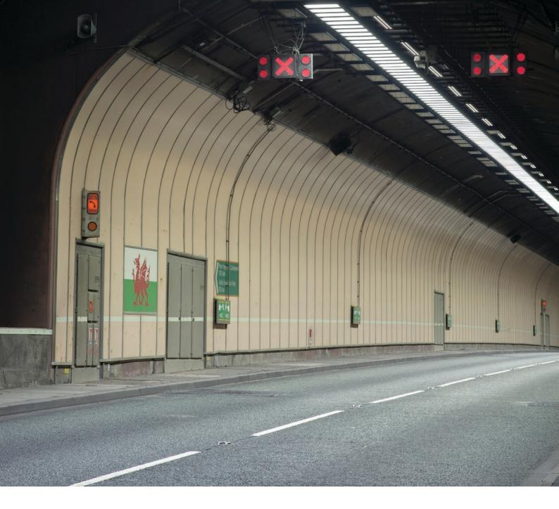
The A55 Penmaenbach tunnel in particular, also required the existing lighting to be retained until the new lighting was installed and commissioned. This was because the tunnel needed to be opened for traffic each morning after night-time refurbishment work.
