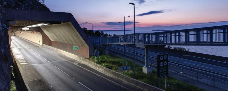
External photometers continually monitor these daylight levels and feed brightness data to the lighting controls, which instantaneously determine the correct corresponding lighting required within the tunnel.
