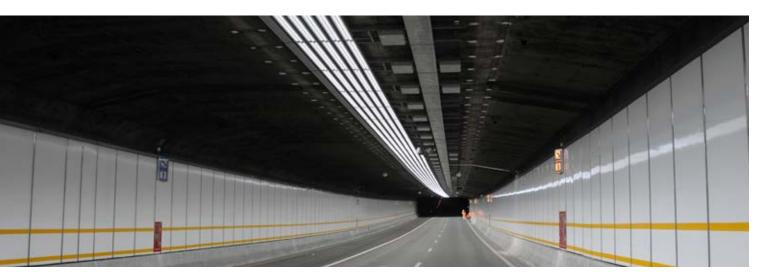
The superior color rendering and higher perceived brightness makes it easier to distinguish objects and shapes. Drivers detect movement faster and from a greater distance with white light, giving them more time to react should the unexpected happen.
