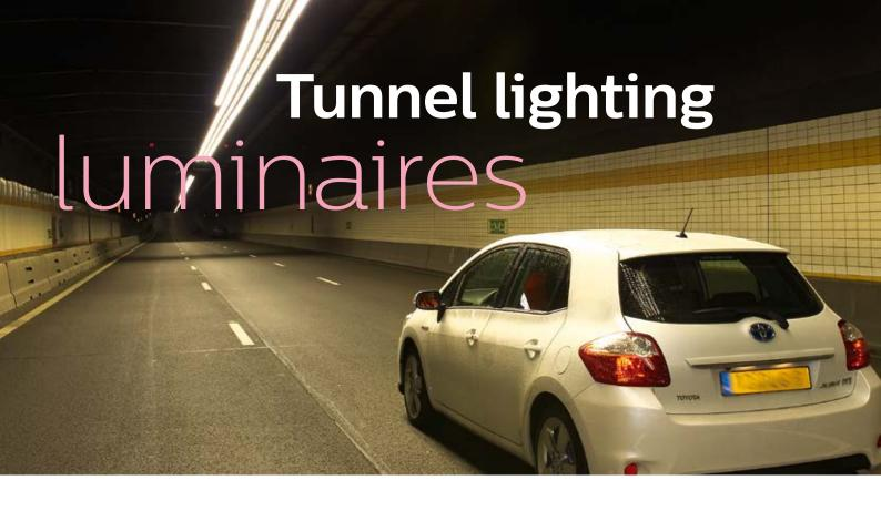
Each zone within a tunnel has its own requirements in terms of lighting design and performance. For example, tunnel entrances require high levels of light with little or no luminaire spacing. In contrast, the lighting in the tunnel interior should be a low level with or without luminaire spacing. With our extensive portfolio of luminaires we can create any lighting concept to provide exactly the right balance between visibility, safety and costs.
