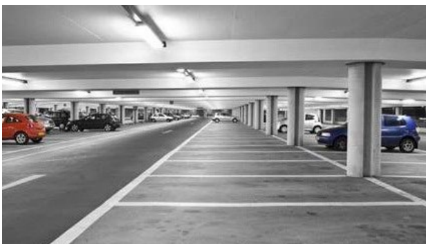
Left picture: CoreLine 'blanket of light' in a parking garage by the wide beam. Right picture: Insufficient light and dark spots as a result of replacing conventional luminaires by luminaires with a lambertian beam.
