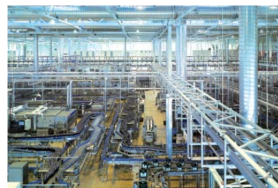
03. Production area medium/ high ceiling 6 to 12 meters
