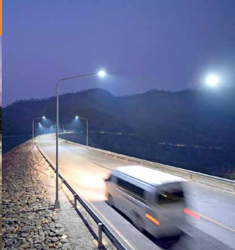
Streetlight for roads
