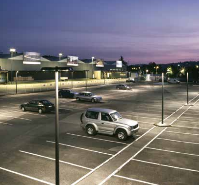
Flood light for carpark
