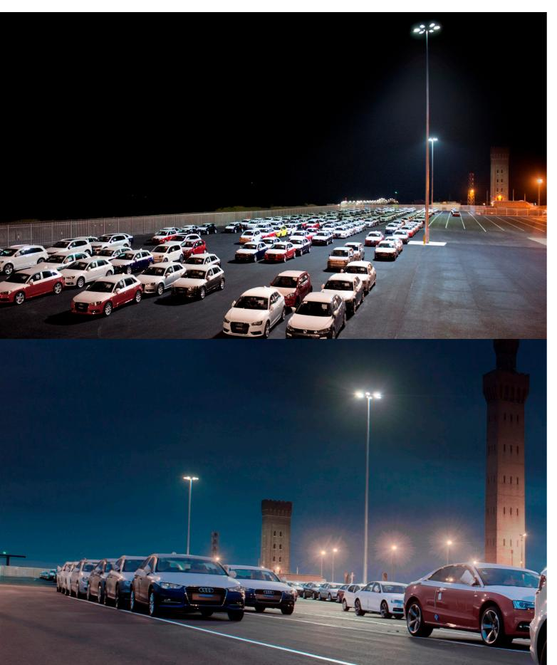
Superior colour rendering and the luminaire's white light, perceived as being brighter and more natural when compared to yellow light, has increased visibility thereby creating a safer working environment.
