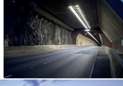
External photometers continually monitor these daylight levels and feed brightness data to the lighting controls, which instantaneously determine the correct corresponding lighting required within the tunnel.
