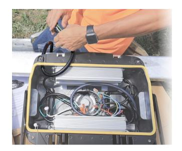
• Attach all Kellem Grip Drop Cables to the Strain Relief Clips located above each Distribution Box at Pole Base.
