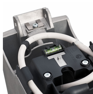
In the case of side-entry mounting, the bubble level ensures that the luminaire is installed horizontally
