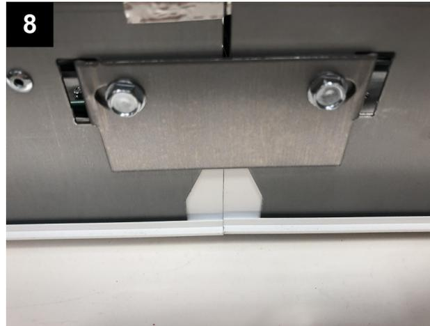
Attach and secure joiner brackets as per supplied TruGroove recessed micro drywall installation instructions.
