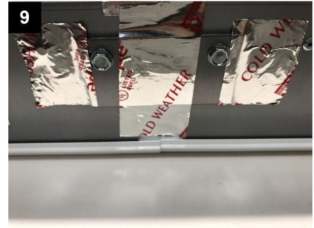
Using supplied tape, seal joint gaps on all sides as shown above.
