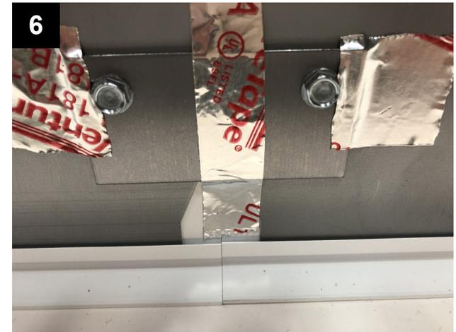
Attach and secure joiner brackets as per supplied TruGroove recessed micro drywall installation instructions. Using supplied tape, seal joint gaps on all sides as shown above.
