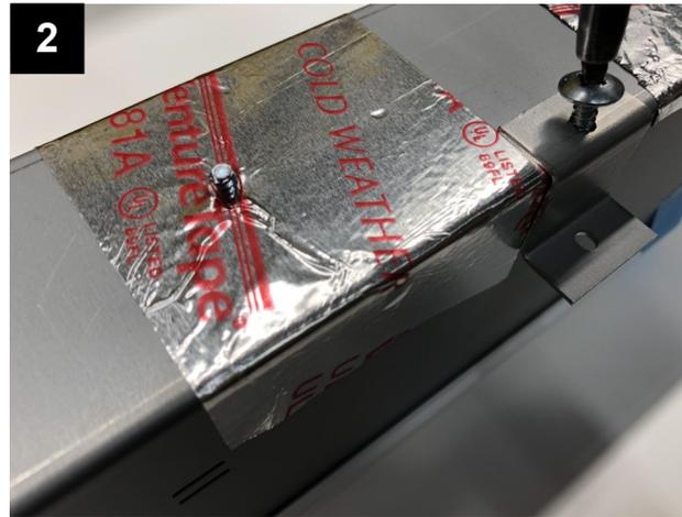
Secure bracket using supplied screw at each location.
