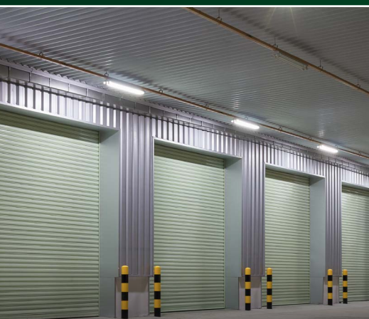
Under canopy lighting
