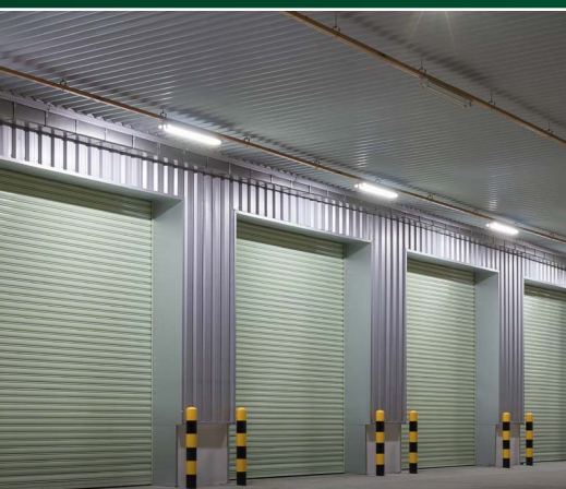
Under canopy lighting
