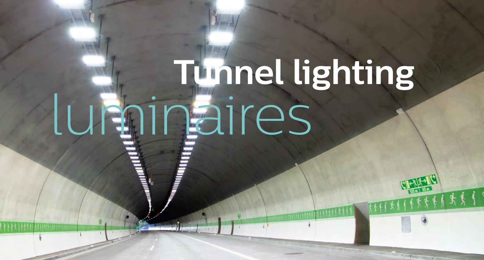
Each zone within a tunnel has its own requirements in terms of lighting design and performance. For example, tunnel entrances require high levels of light with little or no luminaire spacing. In contrast, the lighting in the tunnel interior should be a low level with or without luminaire spacing. With our extensive portfolio of luminaires we can create any lighting concept to provide exactly the right balance between visibility, safety and costs.
