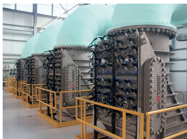
Figure 21. UV drinking water plant.
