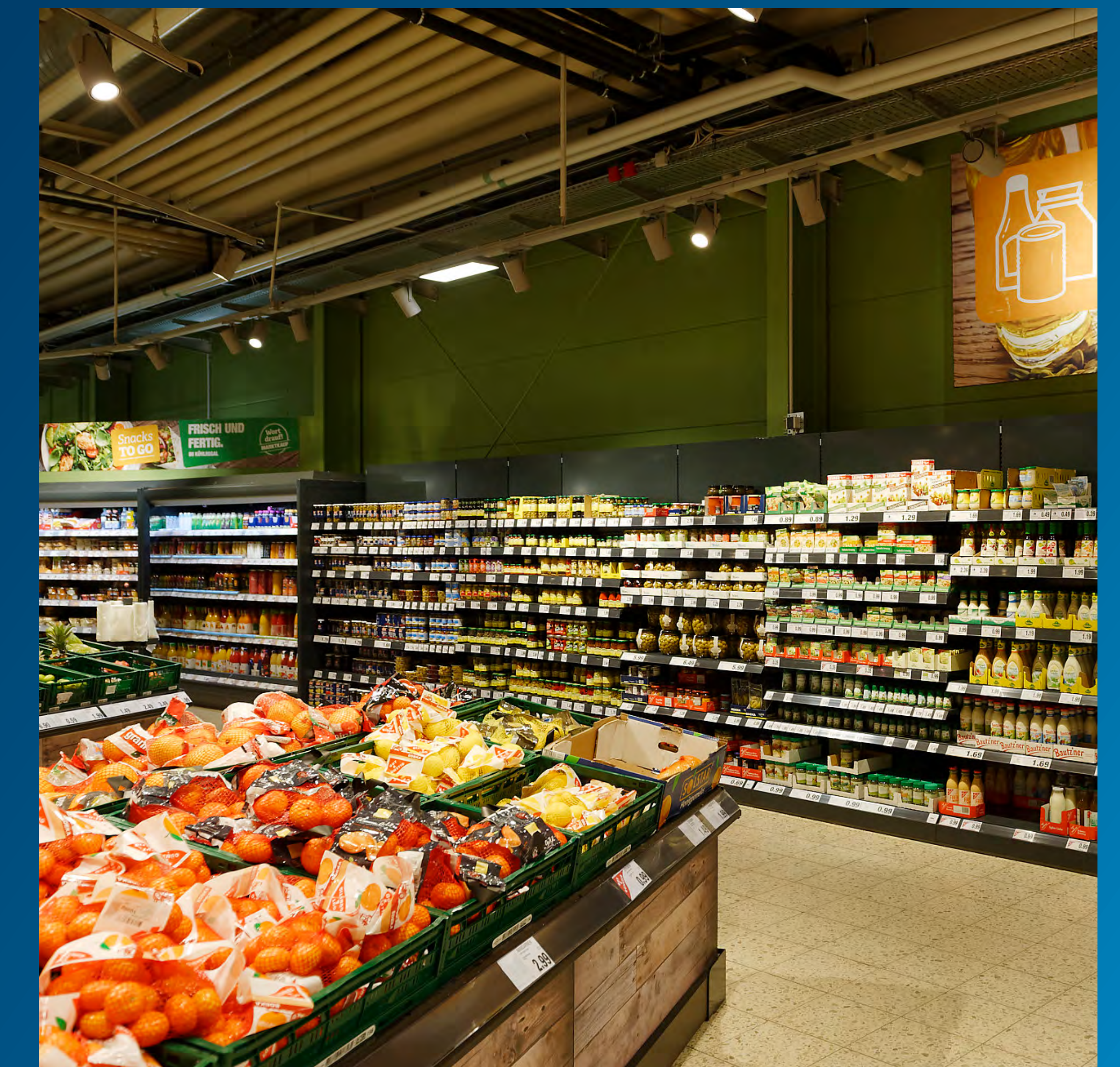
StoreSet Evo used to illuminate the periphery, creating a spacious store atmosphere.
