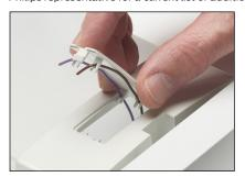
Step 1: EvoKit click SR is shipped with a plate covering the sensor hole. There are two wires secured to the back of the plate. The plate can be removed before or after you install the EvoKit click SR in the ceiling.
