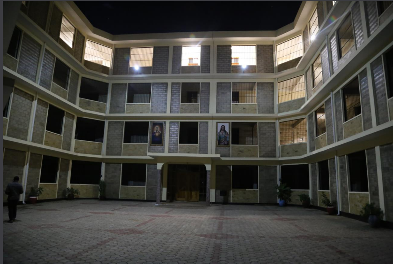
Energy efficient LED battens and solar-powered street lighting for a vocational training center in Tanzania
