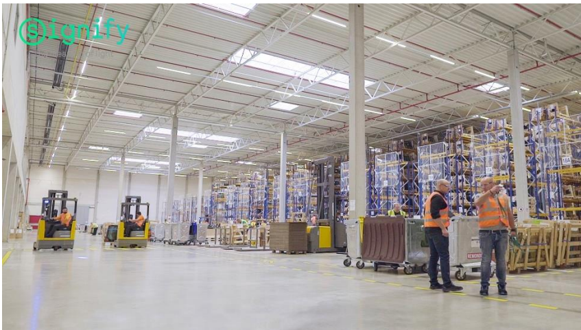
LED lighting installation at NSG Group warehouse
